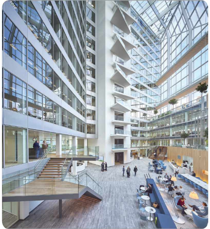
Cool air from the ground floor at The Edge is circulated to the top of the atrium to thermo wheels then released to the outside.
